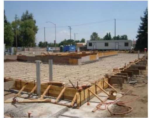
Right: Test and certification building floor prior to concrete pour, July 2006.
